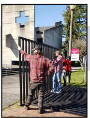
Left: The "cage" pieces around our new furnace unit in the courtyard have now been installed, and the chain link fence units removed. Below: The final cage at last! The Wells Hall HVAC system is complete.
